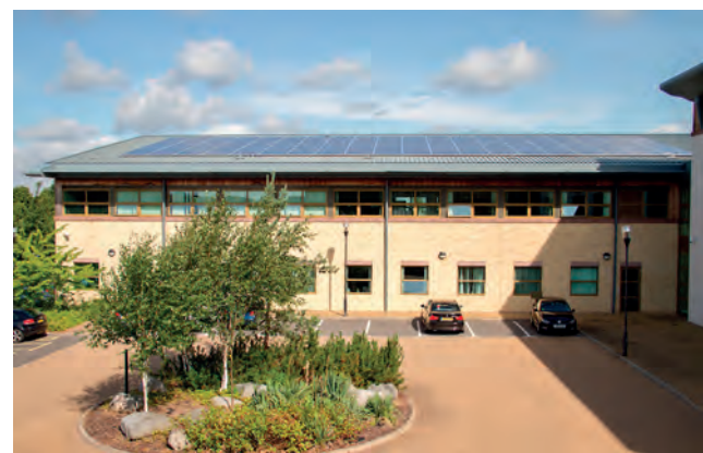
Time team: Evo Energy's installation team worked around Centre Parcs HQ's operational needs to minimise disruption and complete the 50kWp project in just one week
