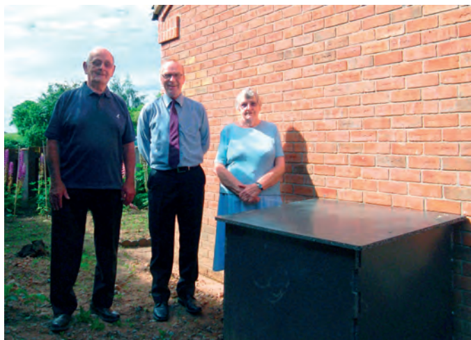
Well grounded: The now defunct RHPP created an opportunity for Shropshire Rural Housing Association to efficiently and cost-effectively transform the heating for tenants in a third of their housing stock
