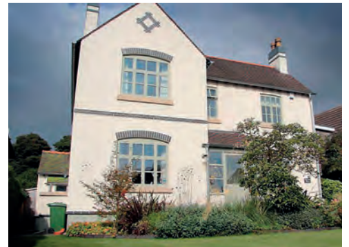
Trend setters: The Engelke family's Wolverhampton home has become the first in the UK to benefit from Viessmann's new Vitocalor 300-P fuel cell
