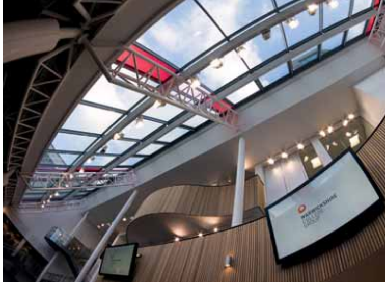
Learning curve: Royal Leamington Spa College's £12m redevelopment boasts a plethora of energy saving technologies including LED lighting, insulated cladding and ASHPs
