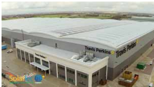
Cashing in: Travis Perkins' 157.5kW PV system at its Warrington regional distribution centre is expected to yield combined FiT income and bill savings of almost £1m over 25 years
