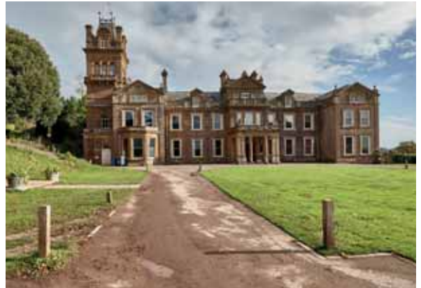
Pipedream: Hestercombe House, Somerset, has ditched an ageing 60kW oil fired boiler for a biomass district heating system, utilising pipework from REHAU
