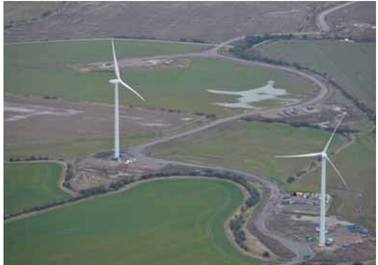
Close proximity: The potential for flooding is significant as RWE npower's 20.5MW Essex windfarm, sited just 300m from the North Sea
