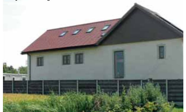
Final straw: Chris Gibbins has achieved zero carbon living by building his house with straw bales, and using an Ecodan ASHP for space heating and hot water
