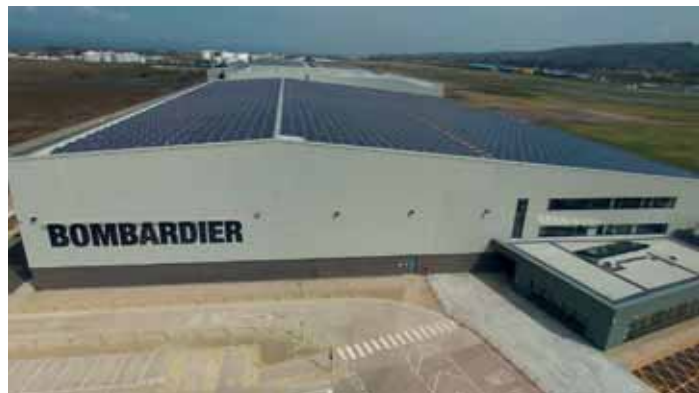
Winging it: Bombardier's 14,000 panel 3.6MW PV array at Belfast City Airport is the largest solar system in Ireland
