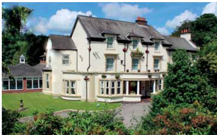
Hot property: A 180kW cascade biomass system from Windhager is meeting the entire heating needs of the 25 bedroom Briars Hall Country House Hotel
