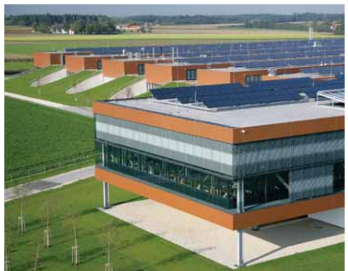
Leading by example: Fronius powers its production site in Austria using its own PV system
