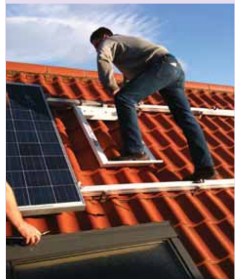
Step by step: Greenfix's solar safety step means no more broken tiles or tools slipping off the roof
