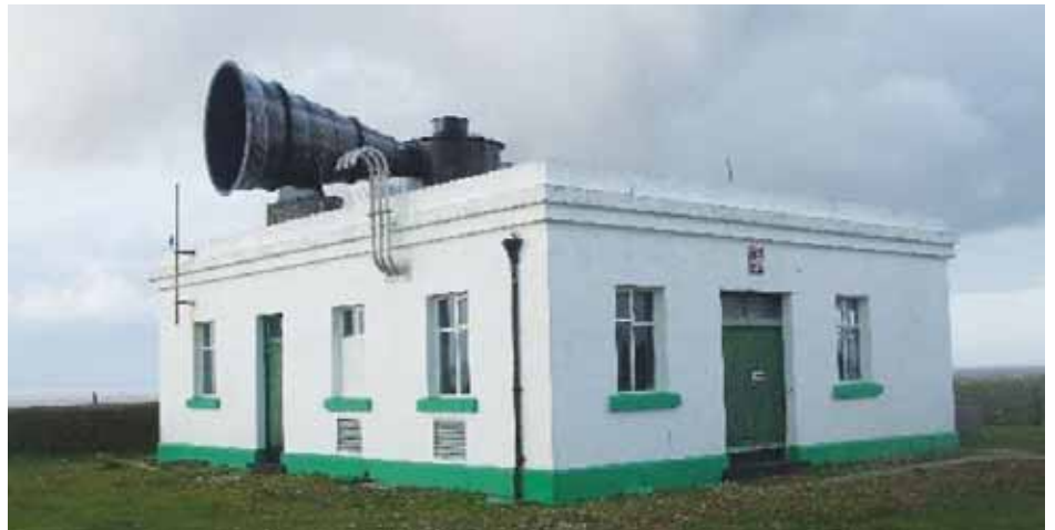
Loud and clear: Navitas installed a biomass system at Fog Horn Keepers Cottage, in the Bristol Channel
