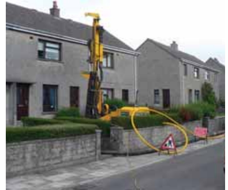
Northern light: Rocklift installing GSHP boreholes on the Orkney Islands
