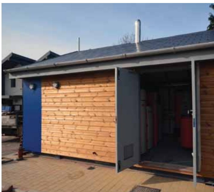
Room mate: Windhager's BioCABIN, a pre-packaged plant room for larger biomass heating installations
