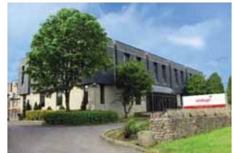
Branching out: Windhager UK's new headquarters at Marshfield, Gloucestershire, features a showroom for the company's range of biomass technology
