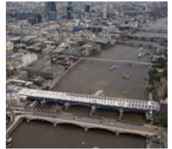
Trail blazing: The installation of London's largest solar array above Blackfriars Railway Station is scheduled for completion later in the year
