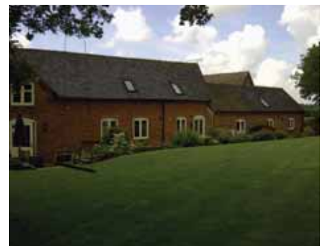
Saving the pennies: Sue Wroe says bills for her Derbyshire barn conversion are down 30 percent following the installation of a hybrid system
