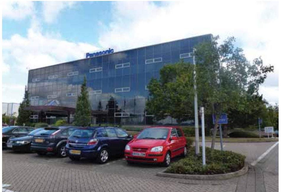
Crowning glory: Panasonic's head office in Bracknell is home to the company's PRO Academy for installers and now a 49.9kWp PV rooftop system
