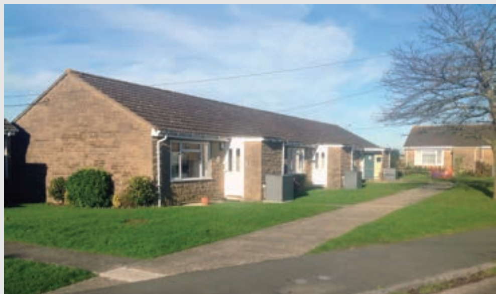
Ground force: Heat pumps located in grey enclosures provide year round heat to the elderly residents at Yarlington, Somerset
