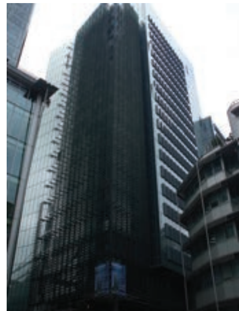
Tube journey: Ropemaker, Ropemaker Place, London has 60 m 2 Viessmann solar vacuum tubes to provide renewable heat for water in kitchens, washrooms and showers
