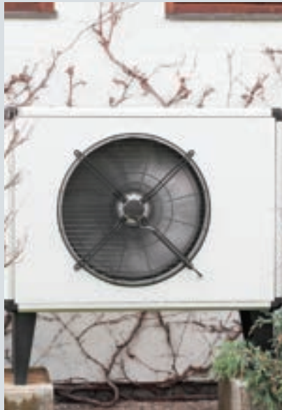
Fall back: Air source heat pumps have a higher requirement for bivalent energy than their ground source counterparts, says Bob Long
