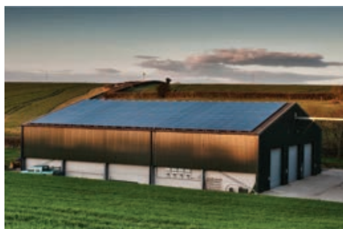
Twilight saga: According to Solar Frontier, high yielding CIS thin film modules are well suited to UK weather, roofs affected by partial shading and low light conditions
