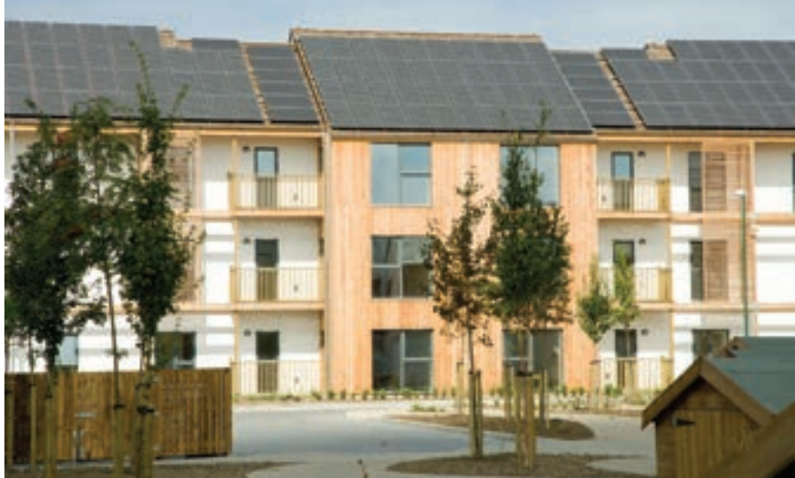
Quality street: Sinclair Meadows, Tyneside, has become the first carbon negative social housing development in the UK by incorporating a commercial-sized PV array
