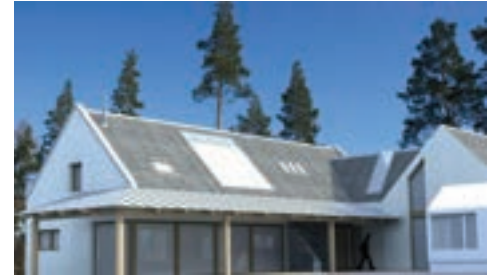
Aberdeenshire architect Ian MacDonald has used wood fibre insulation, triple glazed windows, solar panels and wood pellet boiler to create a low carbon home for his family
