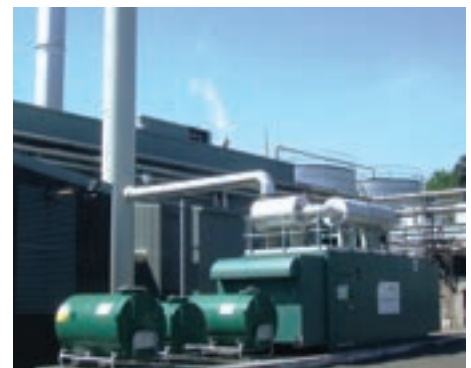
High spirits: North British Distillery's £6m AD unit not only produces clean energy but also processes a third of liquid by-products from the site
