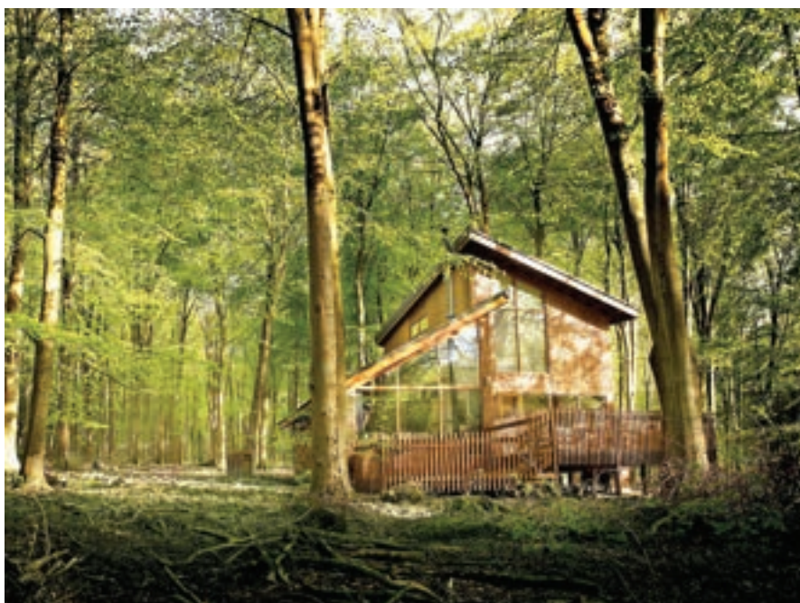
Branching out: All 60 cabins at Forest Holidays, Hampshire, have underfloor heating driven by the Torrent GreenHeat thermal store which also delivers mains pressure hot water.
