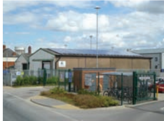
Bright idea: Enphase microinverters were combined with a 19.5kW commercial installation in Goole to overcome variable shading
