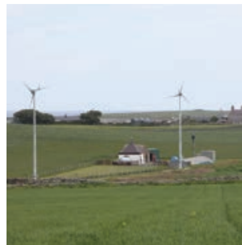
Absolute power: Evance says its Grid+ system enables maximum energy capture whilst allowing only 3.68kW to be transferred to the island of Stronsay's limited grid connection
