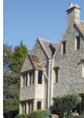
Looking good: Windhager UK BioWIN wood pellet boilers now supply heating and hot water for the manor house, estate cottage, stables and swimming pool at an attractive Cotswolds Grade II listed property
