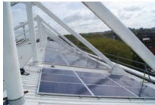
Energy kick: Northampton Saints Rugby Club has boosted its green credentials with a 50kWp array at the club's Franklin's Gardens Stadium
