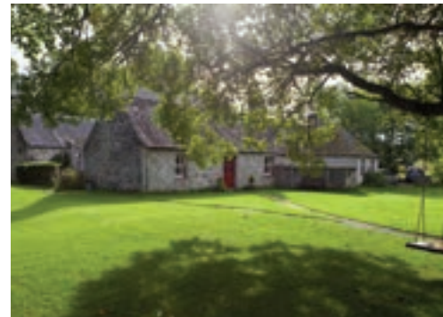
Double appeal: The installation of biomass technology has considerably improved the green credentials of The Dell of Abernethy family home and holiday cottages as well as reducing its energy costs
