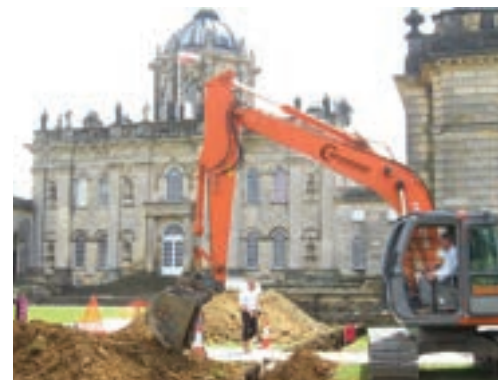
Historic move: The owners of Castle Howard report a £66,000 reduction in annual heating bills since swapping oil-fired heating for a water source heat pump
