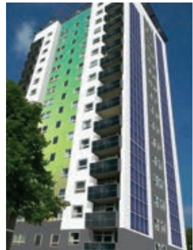
High and mighty: Walsall Housing Group's 65 flat Austin House is the UK's first tower block to be exclusively heated by GSHPs, according to Dimplex
