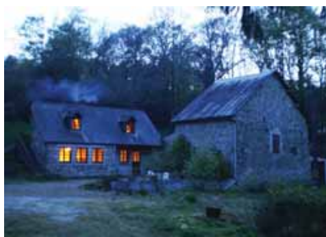
Country life: David and Pam Marchant turned to the Xcel HEATBANK thermal storage unit to facilitate hot water and space heating throughout their rural property via wood burning stoves
