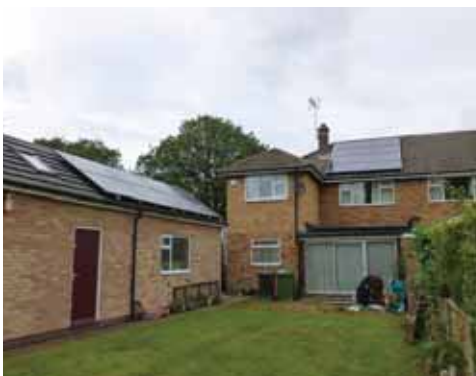
Problem solving: Electrical engineer Allan Davis turned to Enphase microinverters to overcome shading issues for his 4kW split roof PV array
