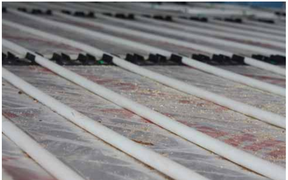
Looking ahead: Although an effective way to secure future business, making UFH compatible with the introduction of a heat pump at a later date requires an experienced system designer
