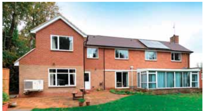
Doubling up: Surplus energy generated by the solar PV is fed to an ASHP at this home in Warwickshire to further lower its energy consumption and carbon footprint
