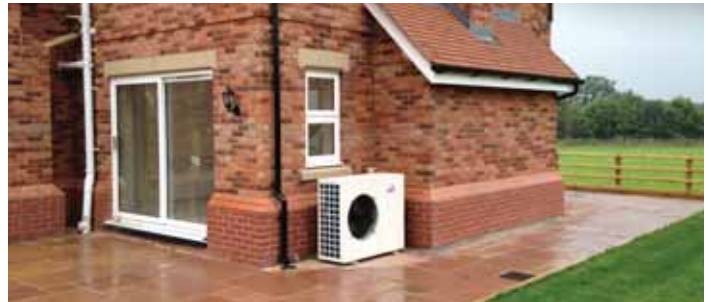
Cool reception: Husky Heat Pumps' Alan Dunn advises against specifying high temperature heat pumps due to significant extra running costs
