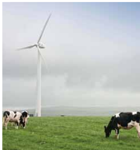
Generation game: The Endurance X29 turbine on Matthew Rowe’s dairy farm at Liskeard in Cornwall is predicted to supply 500,000 kWh a year
