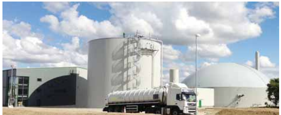
Cooking on gas: Emerald Biogas' new £8m anaerobic digestion facility in County Durham will supply clean electricity to 2000 homes and fertilizer from local food waste
