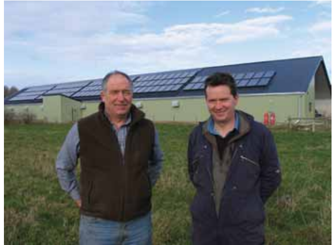
Big deal: Steve and Sam Barker have cut carbon emissions at their Shropshire game rearing company by 34 tonnes per annum with a 194kW solar thermal system
