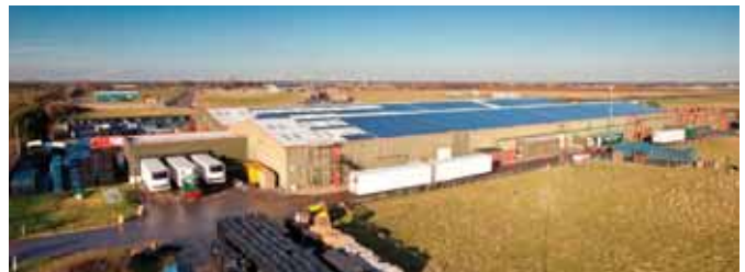
Big money: E Park & Sons' 2,742 panel 681kWp PV system nets the potato producer £100,000 per annum in FiT income and energy savings
