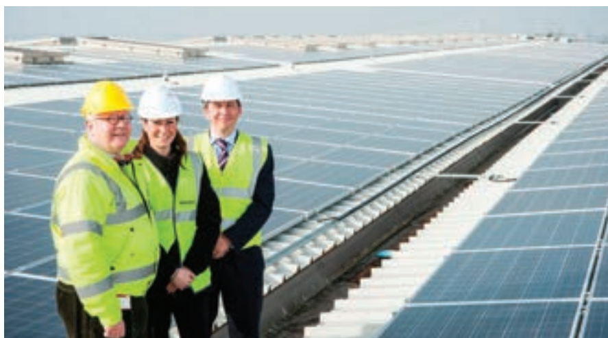
Aiming high: (L-R) Tim Pollard, head of sustainability, Kirsty Greggs, environmental manager, and Simon Allen, renewables director, inspect Wolseley UK's 2MW 8,020 panel PV system
