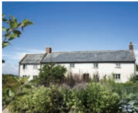
Recipe for success: After suffering devastating fire at the site, TV chef Hugh Fearnley-Whittingstall's River Cottage is now fully heated by biomass
