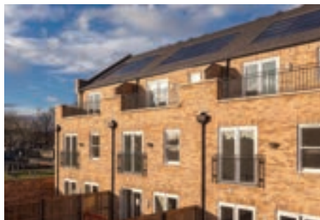
Flagship project: Romag's PV roof tiles were used on the UK's largest zero carbon housing development at Park Dale, in Castleford, West Yorkshire
