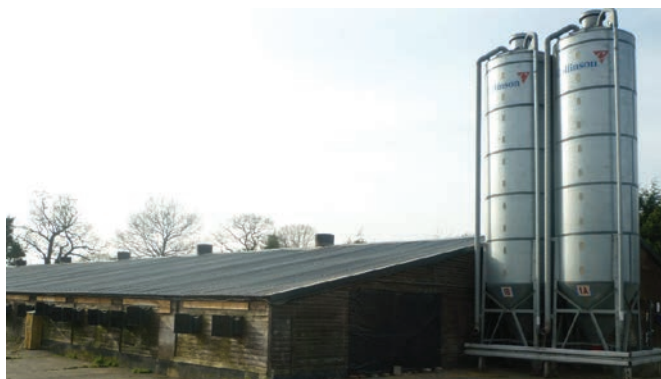
Liquid gold: SA & DE Dixon of Shropshire is the first poultry farm in the UK to be heated by a water source heat pump
