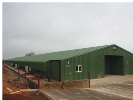
Power cut: Energy consumption during the winter cycle in the poultry sheds at Stonehouse Farm, Gloucestershire, has been cut from 49,000kWh using LPG to only 4,000kWh using six Ecodan ASHPs
