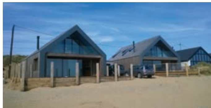
Life's a beach: Heat from bore holes drilled under a beach in Kent now warms these two eco-friendly holiday homes
