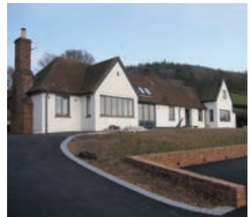
Future proof: A draughty 1930s-built Somerset bungalow has been given a complete makeover including the use of a NIBE GSHP
