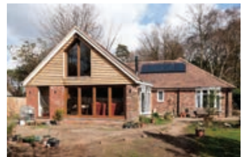
Virgin territory: Surrey-based installers Source Heat Pumps fitted the UK's first domestic NIBE all-in-one hot water, control and buffer store package at the Taylors' renovated bungalow
