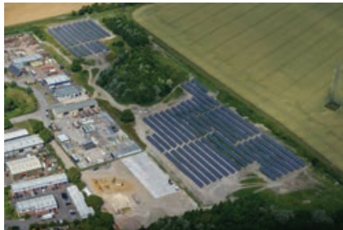
Proceed with caution: Hopton Industrial Estate's solar farm near Devizes had to be designed sympathetically to the surrounding landscape as it is in full view of a nearby Area of Outstanding Natural Beauty
