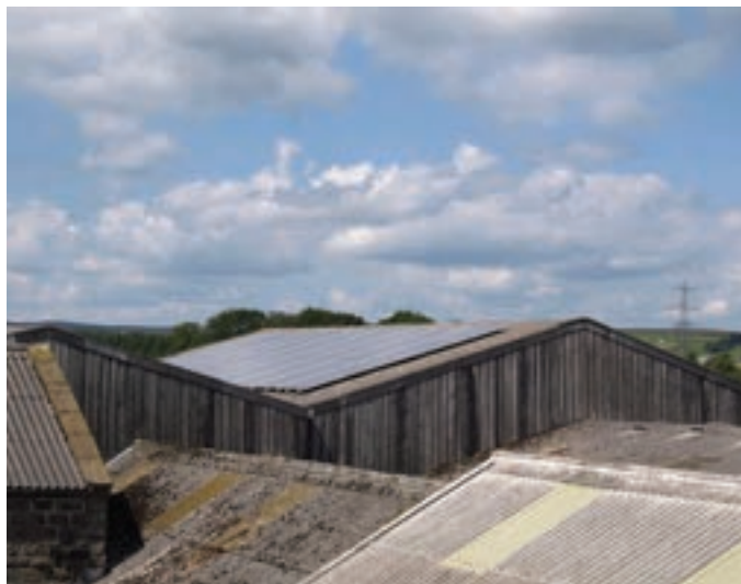
On the map: This year's Tour de France route through Yorkshire took riders passed Norcroft Energy's 18.35kW install at Ranah Stones Farm
