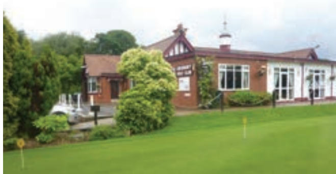
On the green: Didsbury's 18 hole golf course opted for a containerised biomass system to combat rising fossil fuel prices
