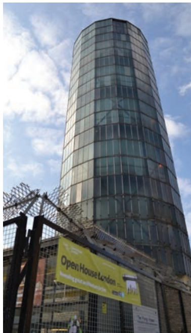
Dizzy heights: PDHU's accumulator tower has provided district heating for over 3,000 properties in Westminster for over 60 years
