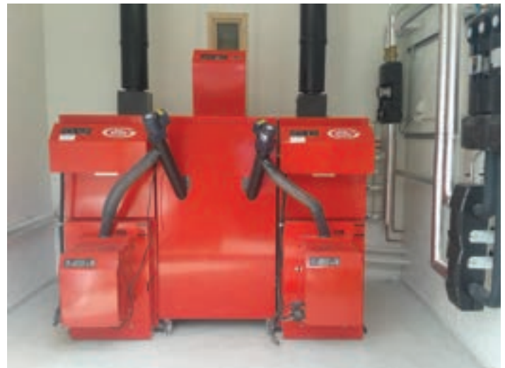
First choice: The Grant Spira condensing wood pellet boiler was chosen by Hull-based installer Leighton's due to its impressive efficiency
