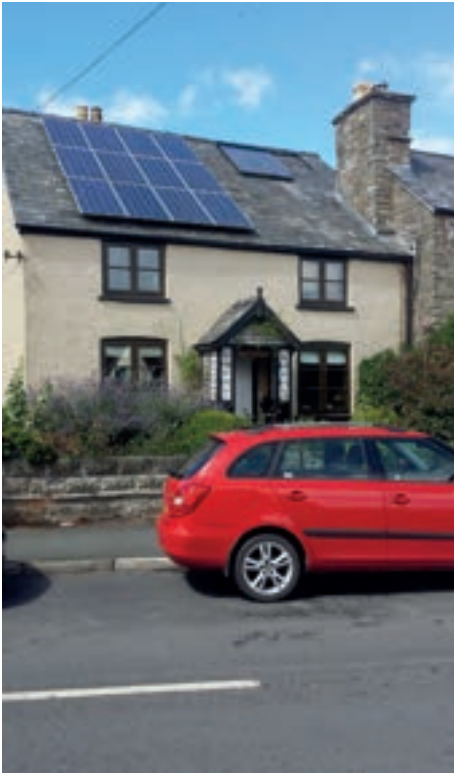
Solar thermal technology sharing roofspace with PV on a house in the UK
