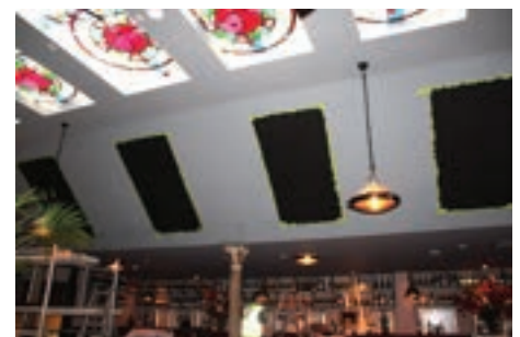
6 Awaiting decorative layer of paint
