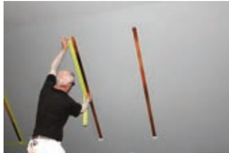
1 Preparing for the coating
