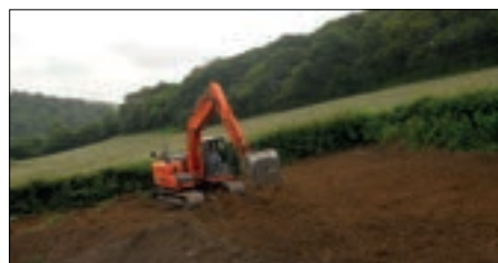
Top: The living area of the beautifully restored 17th century church. Middle left and right: Preparing the underfloor insulation. Bottom left: The project began with the digging of a 50m trench for the heat pump
