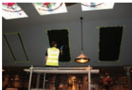
5 Applying the second coat
