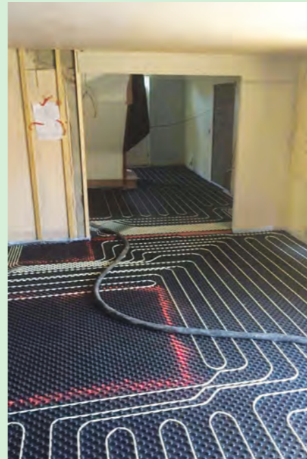
Above: Preparing the underfloor heating
