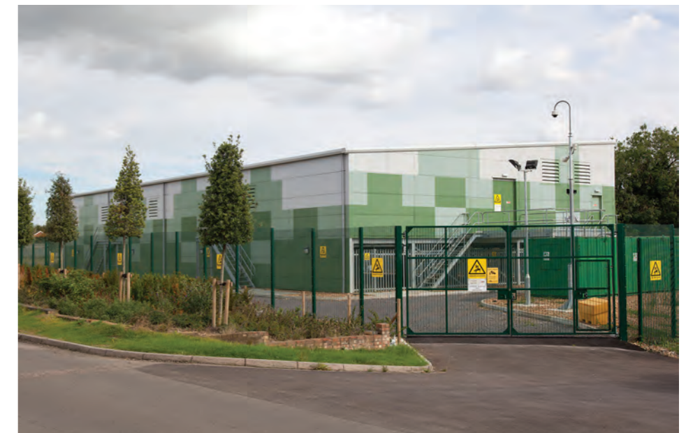
Top: The 'big battery' trial at UK Power Networks. Below: The company's test facility at Leighton Buzzard, Bedfordshire
